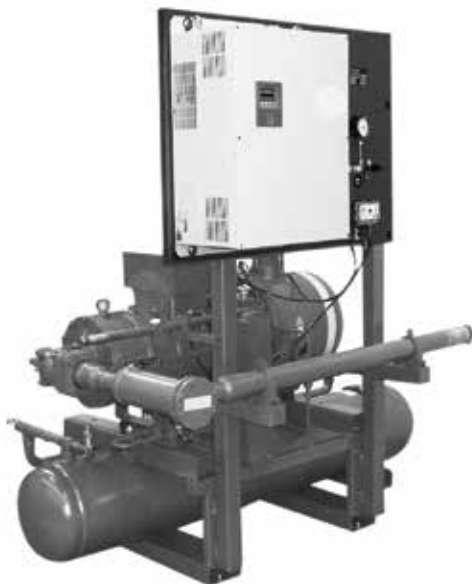
CX-Series Screw-Pack (Fitted with VSD Inverter)
